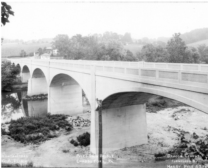
Twin Bridges 1927. The bridge and the location derived its name from two original covered bridges which spanned the Brandywine. Photo Courtesy Chadds Ford Historical Society
